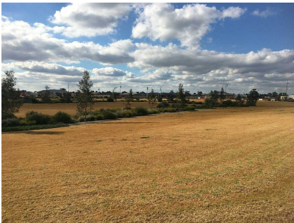
Figure 12 Example vegetated detention basin with maintained kikuyu grass cover (Parkview Estate, Echuca)
