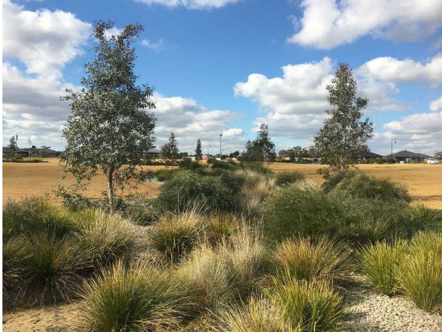
Plate 1 Parkview Estate (Echuca) vegetated swale (~2 years established)
