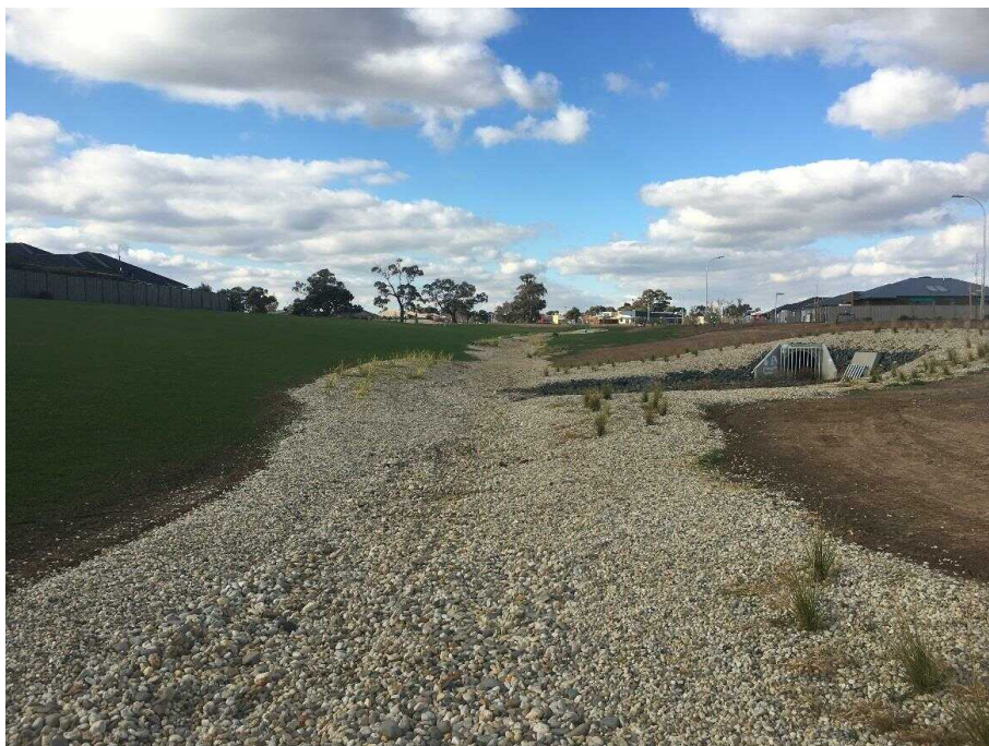
Plate 2 Murray Gardens Estate (Echuca) vegetated swale (~3 months established)
