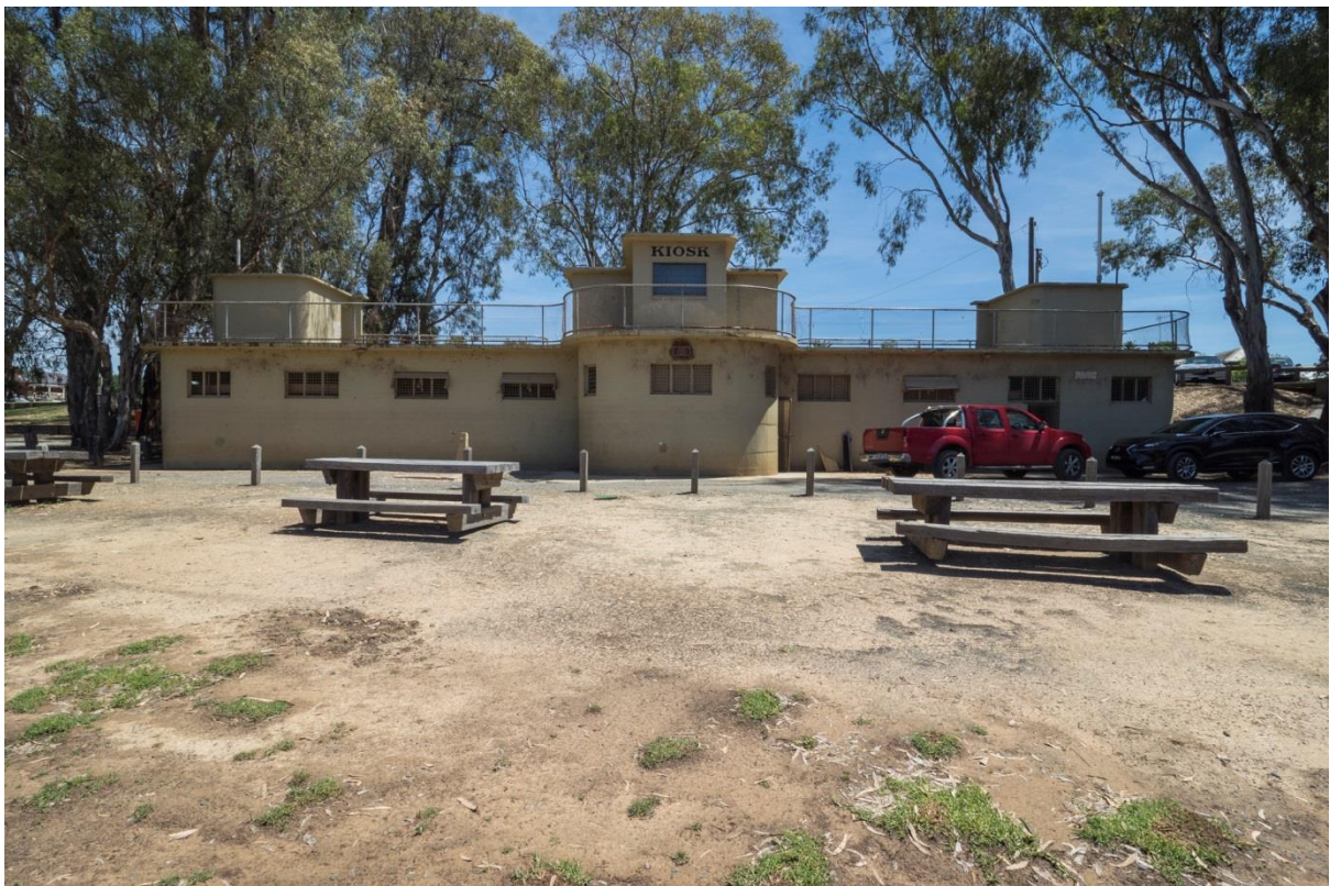
Plate 4: Concrete pavilion, containing changing rooms and kiosk facing west.
