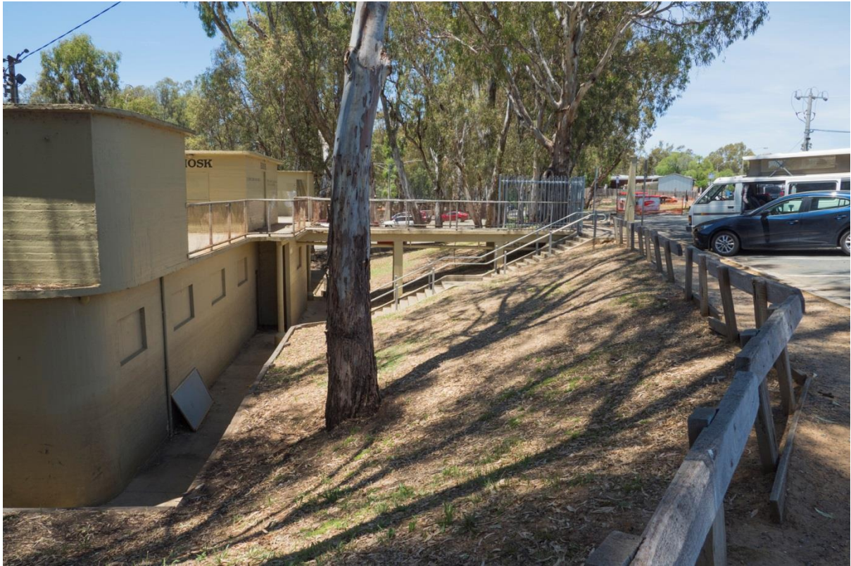
Plate 13: Rear wall of pavilion facing south.
