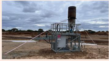
To prepare Council for the EPA mandate of landfill gas capture by 2030 and explore methods of offsetting other emissions – this year we initiated a landfill gas flaring trial at the Moama landfill.
