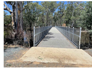
Existing boardwalk to be protected and retained
