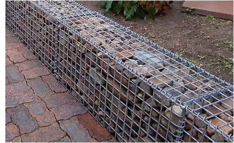
Gabion retaining wall
