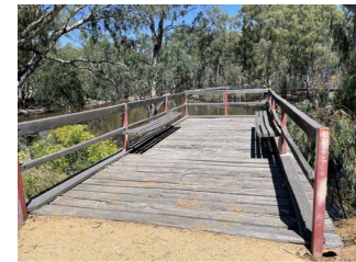
Existing viewing platform to be protected and retained
