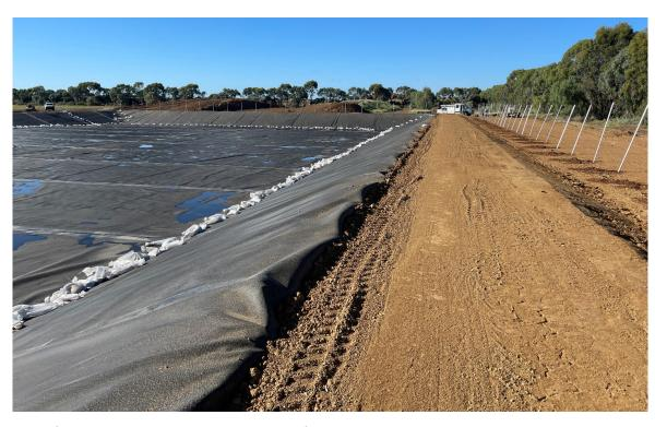
Security fencing installation around the completed landfill leachate pond.
