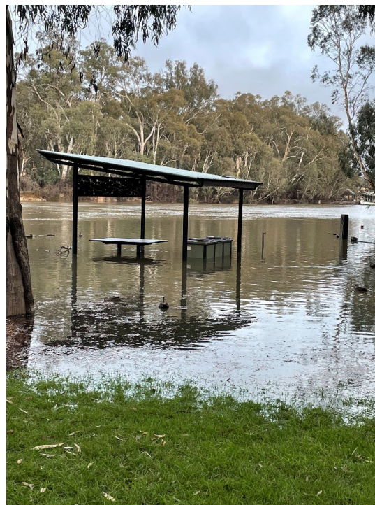
Moama Beach Flooding
