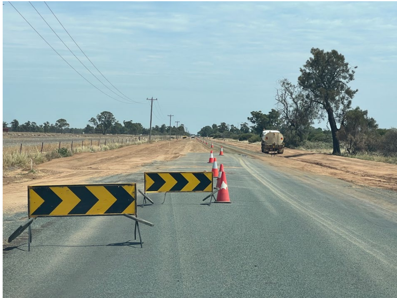
Works on Bunnaloo Road.
