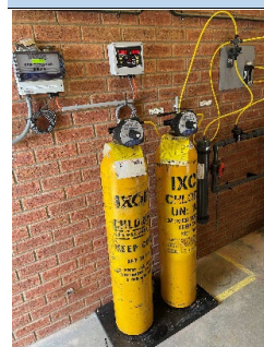
Barham chlorine gas dosing replacement
