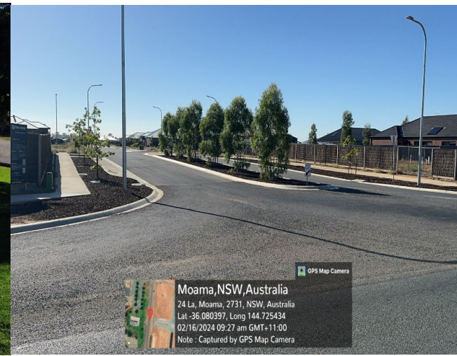
The Range Estate Entry- Inspection for handover
