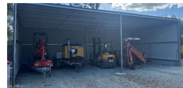
Machinery shed complete for minor plant at Moama WTP.
