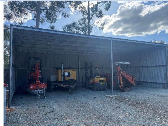
Machinery shed complete for minor plant at Moama WTP.
