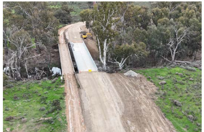
Council put the finishing touches on the Tooranie Road / Yarrein Creek Bridge, marking the final timber bridge on our replacement list.
