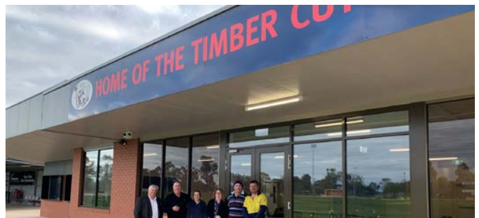
The pavilion underwent renovation and extension works to increase capacity for use
