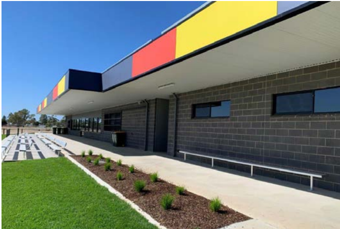
The new multipurpose pavilion has been welcomed by local user groups and visitors
