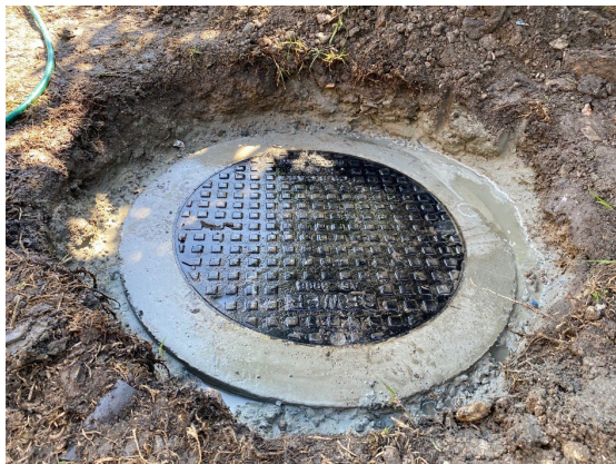
Sewer maintenance hole
