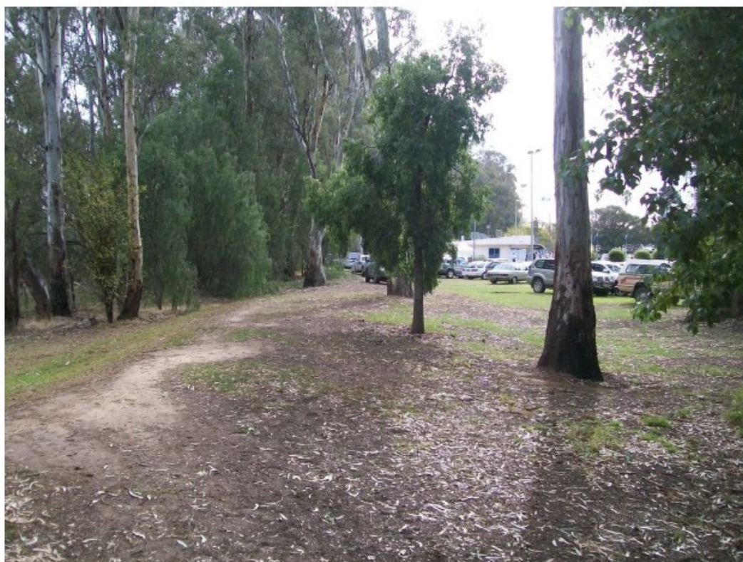
Photograph 1 Town Levee opposite the Bowling Club
