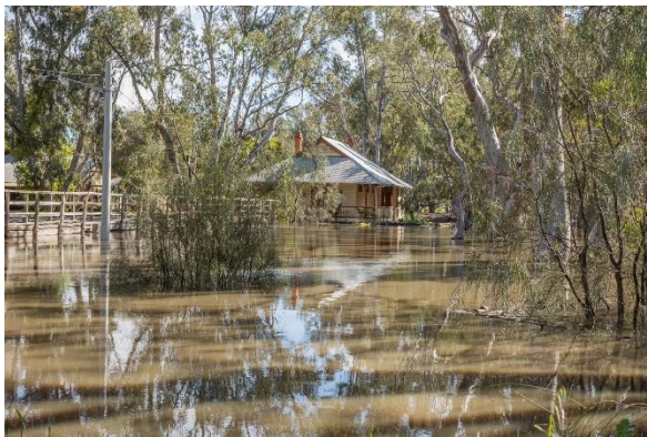
Photo 4-9: 2016 Flood - Old Court House Bridge
