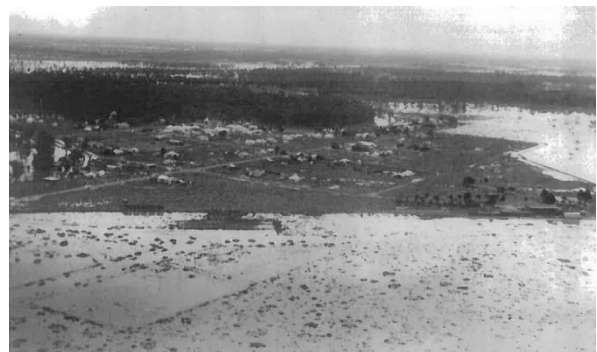
Photo 4-18: 1956 Flood - Moulamein Township Surrounded by Floodwater
