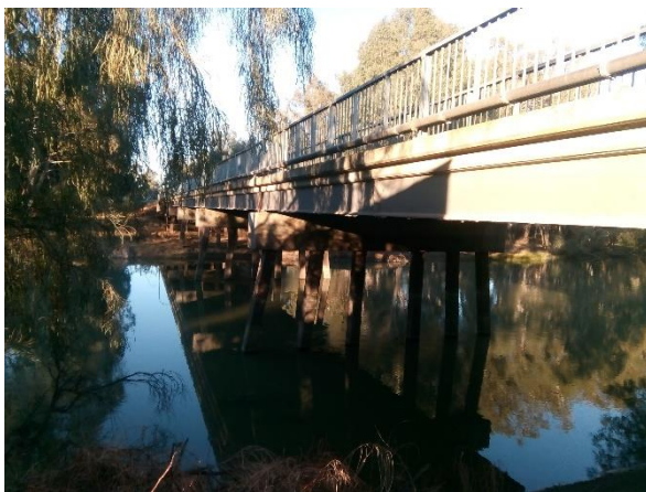
Photo 4-1: Moulamein Road crossing the Edward River
