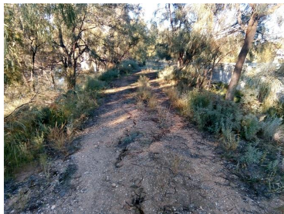
Photo 4-6: Crest of the northern town levee
