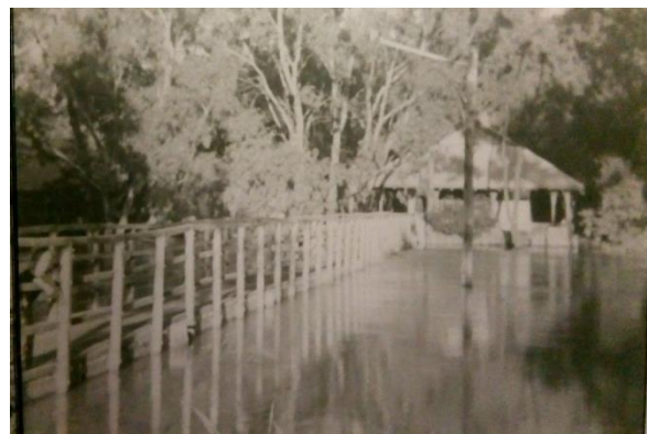
Photo 4-20: 1974 Flood - Old Court House Bridge
