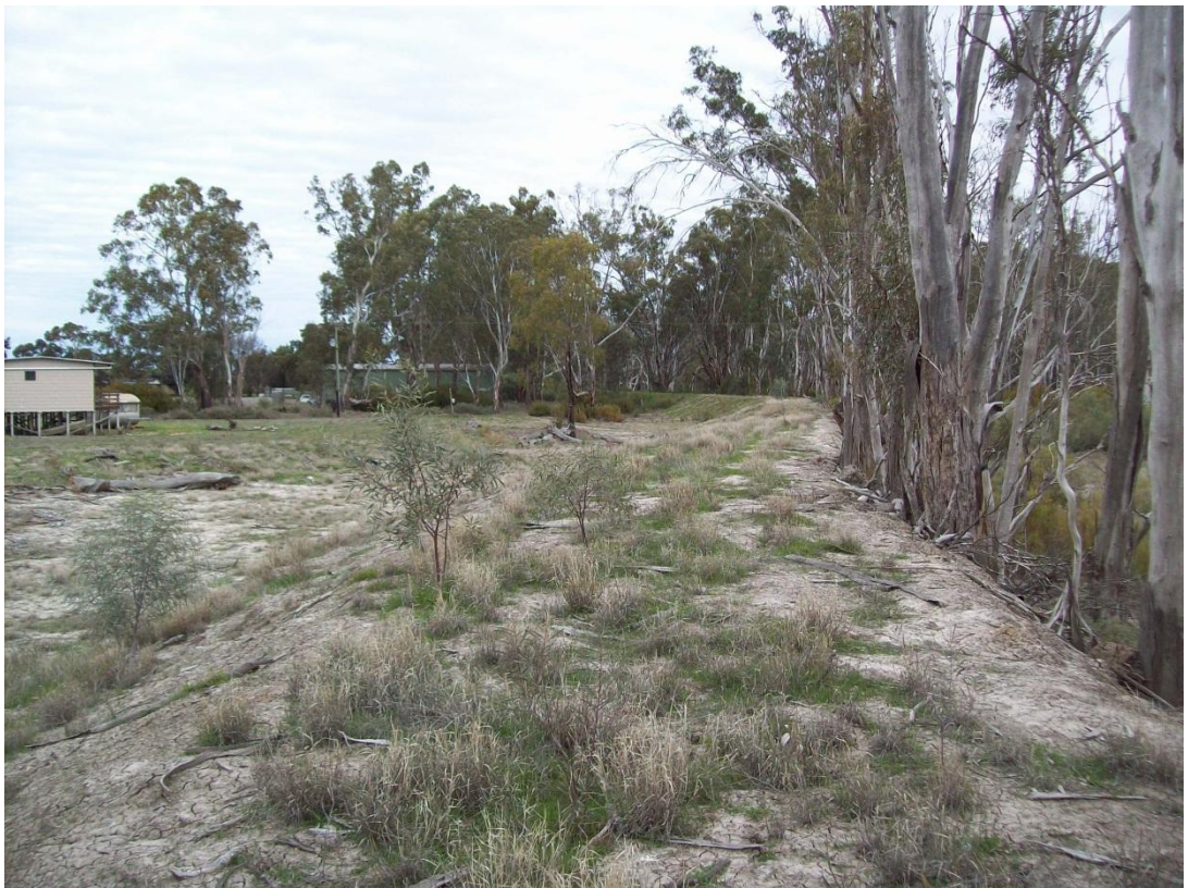
Photograph 4 South side rural levee
