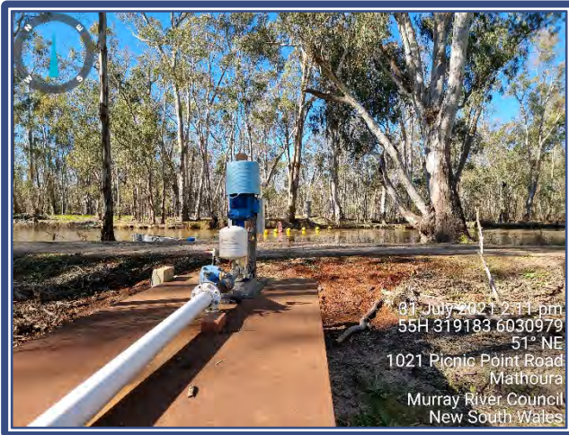
Figure 8-1 Existing pump on platform
