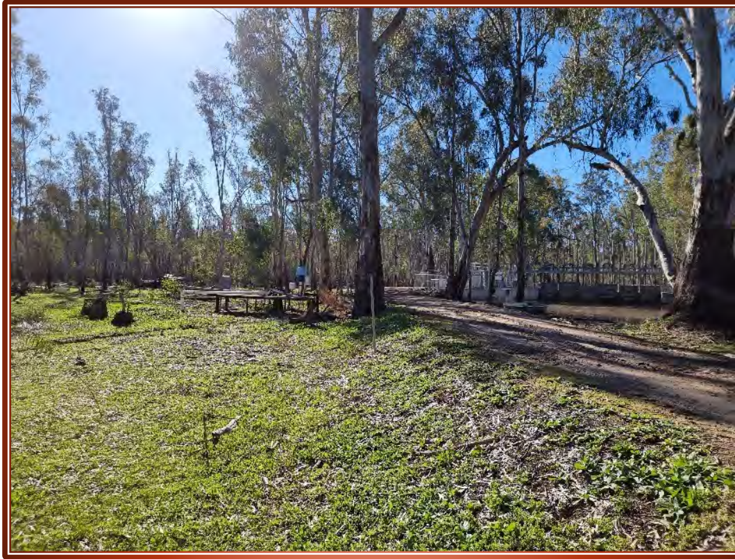
Figure 3-3 Pump site looking downstream with the Edward River Regulator in the background
