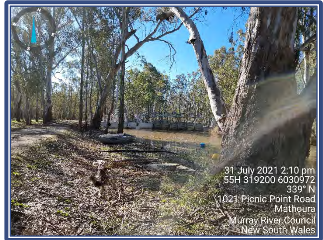
Figure 8-4 View looking Upstream showing suction pipe in River
