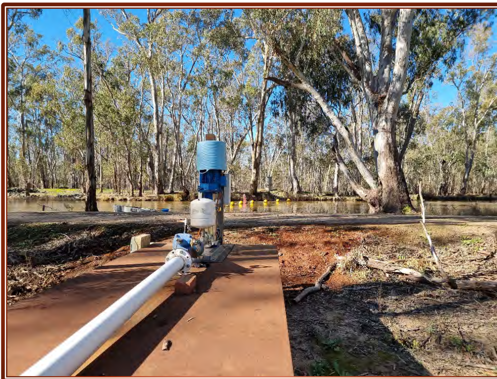
Figure 4-1 - Pump site looking toward Edward River
