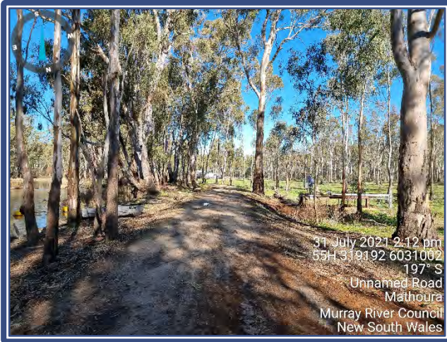
Figure 8-2 – Levee Bank looking downstream with pump on dry side
