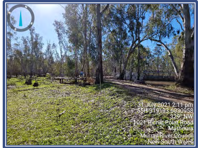
Figure 8-5 View looking upstream with pump on dry side of levee
