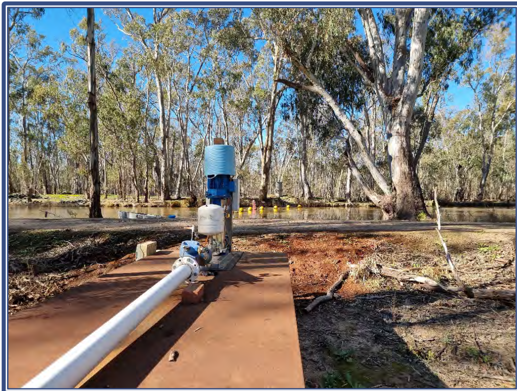
Figure 3-1 Pump Site looking toward Edward River
