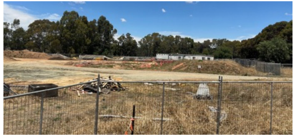
Figure 15 Looking south from building footprint 0 – 5° downslope. Mackenzie Davey 2021
