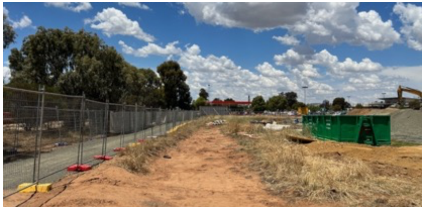
Figure 14 Looking east from building footprint upslope. Mackenzie Davey 2021
