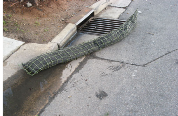
Example – Drain Filtering / Sediment trap
