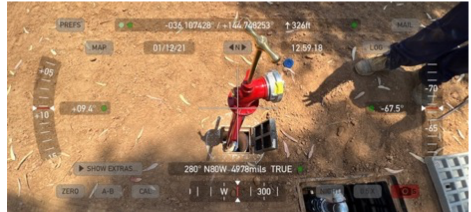
Figure 21 Fire hydrant on Boundary Road see photopoints plan for location. Mackenzie Davey 2021
