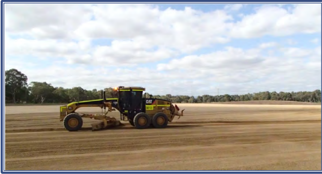
Figure 2-11 - Photos showing an example of hardstand construction (Source: McMahon Services)
