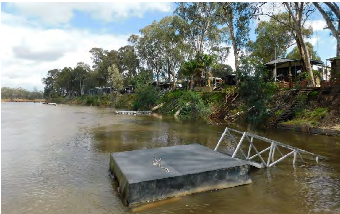
Figure 7 West facing photograph of riverbank and pontoons
