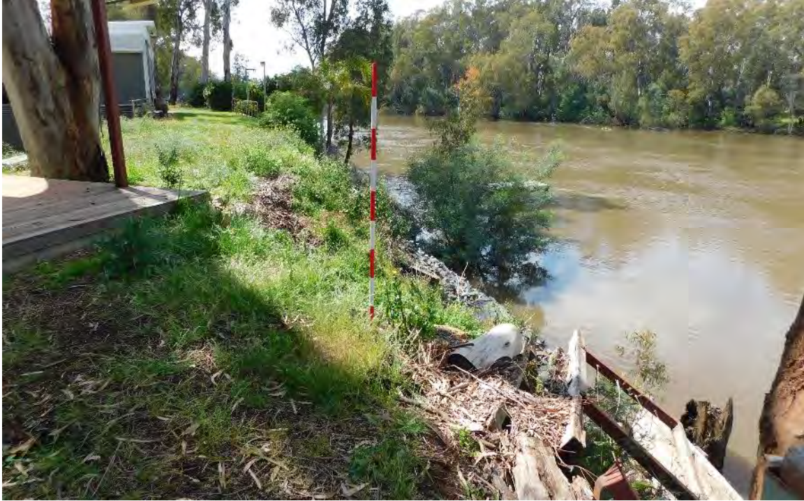
Figure 8 South-west of riverbank with a rock embankment
