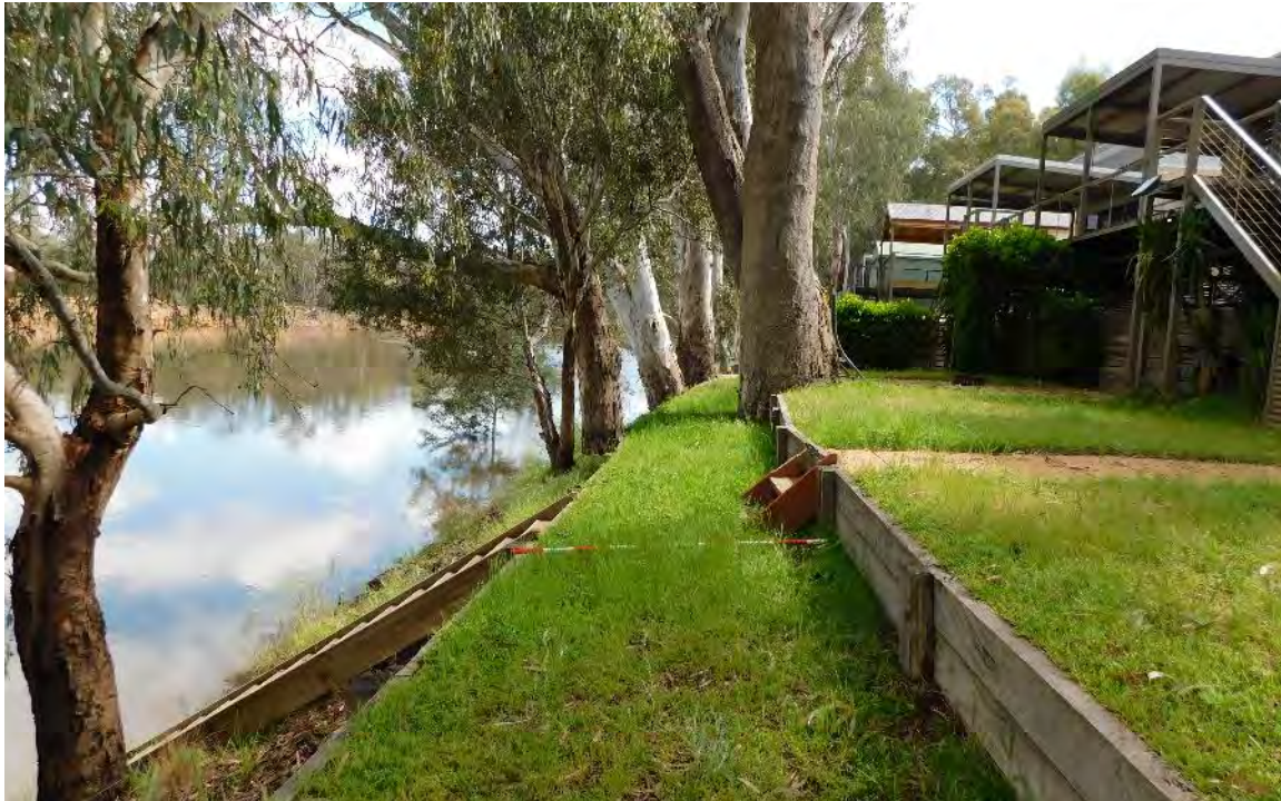
Figure 6 North facing view of disturbance to riverbank
