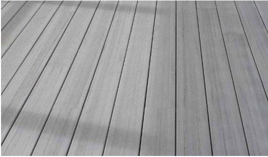
EF-06 TIMBER DECKING 137mm COMPOSITE DECKING BOARD Silver Gum Brushed (Non-Slip) OR SIMILAR
