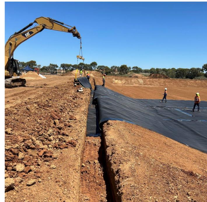
High Density Polyethylene liner being installed into the landfill leachate pond.
