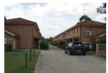
Photo showing poor orientation of building to street with a 'gun-barrel' driveway.
