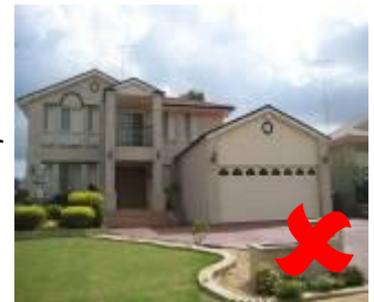
Photo of garage that is not setback to the building line.
