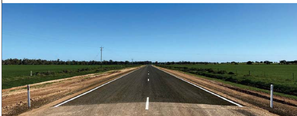
Completed seal at Speewa Road, Speewa.
