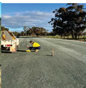
Compaction testing of base layer at Centre Road, Moama
