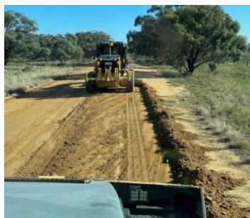
Maintenance grading
