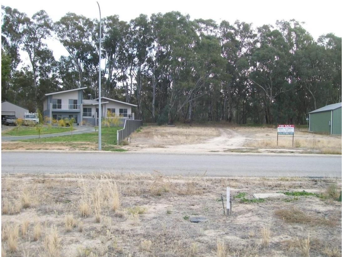
Photograph 2 View from Teddys Place towards constructed levee and river
