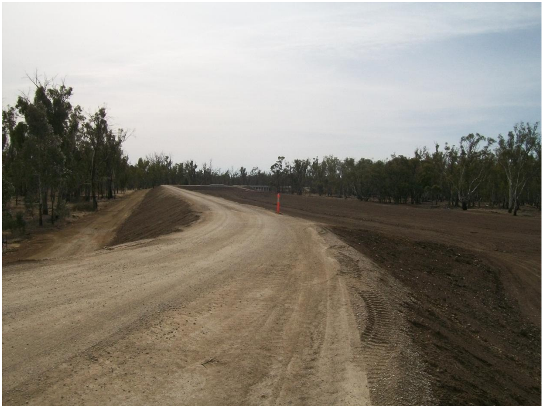
Photograph 4 Koondrook Forest levee bank
