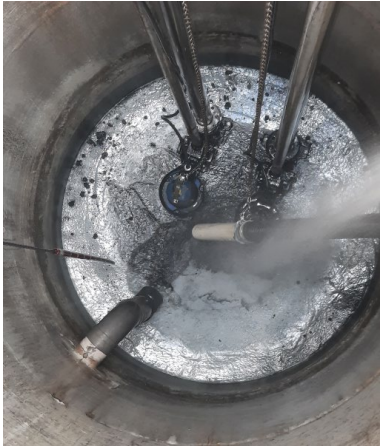
Maintenance cleaning of Moama business park sewer pump station
