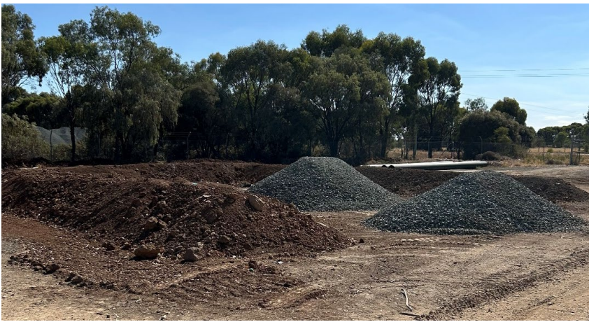
New tyre and mattress drop off bunds are being constructed by the staff to comply with the site Standard Operating Procedure separation distances.
