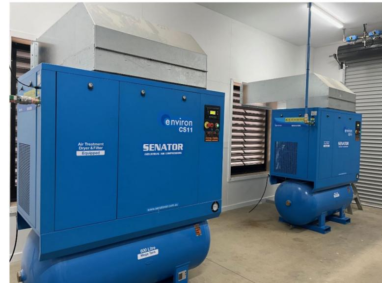
Compressor room housing equipment to operate the singulators and the landfill leachate management system.
