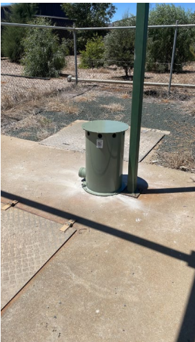
Odour control unit for Sewer pump station in Beer Rd
