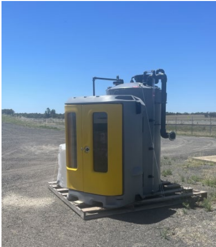
Chemical dosing unit for Wakool WTP
